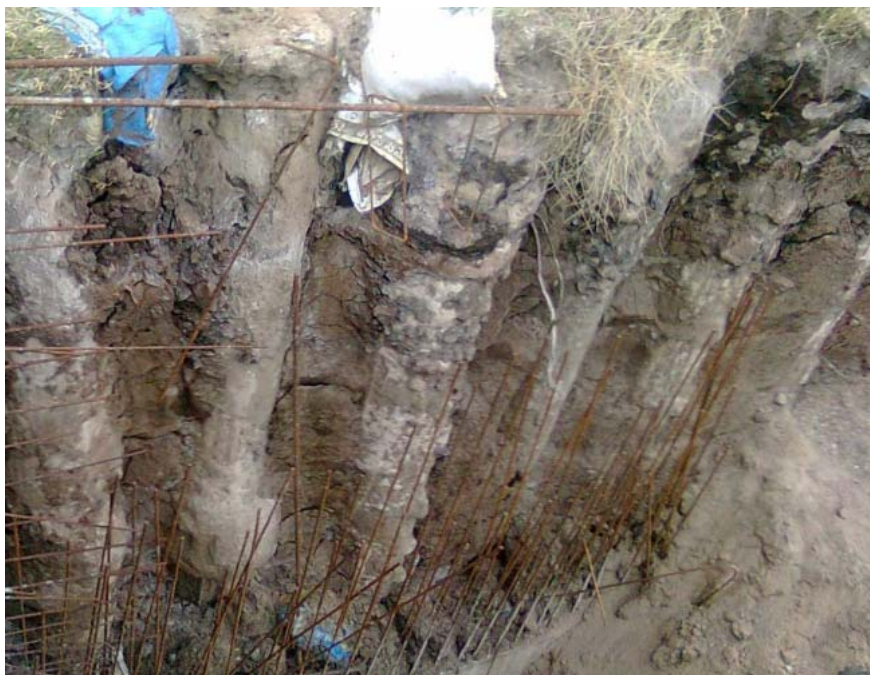
Plate 1. Contiguous Pile Retaining System for Commercial a Complex Vijayawada
